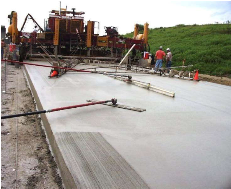
Hand float and straight edge
