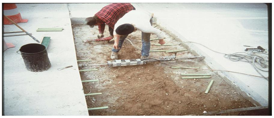
Rams can cause the grout to shoot out which results in insufficient filling of the void.
