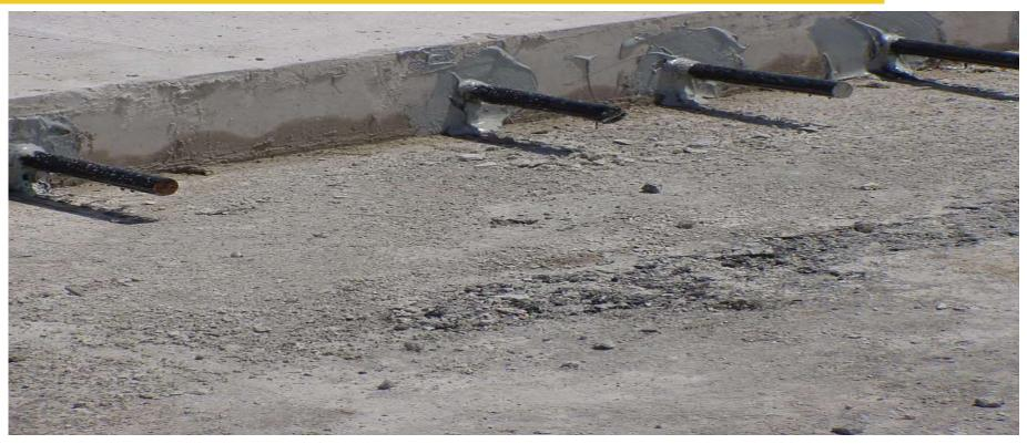
MDOT uses a product called RC250 as a bond breaker to allow the dowels to move freely in the new concrete repair.
